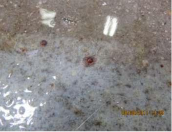
The photos above are of a moisture failure due to the concrete fibers not being properly covered/coated with moisture reduction barrier (MRB). The failure happened within days after installation of the MRB. The floor was not properly burned prior to the installation.
